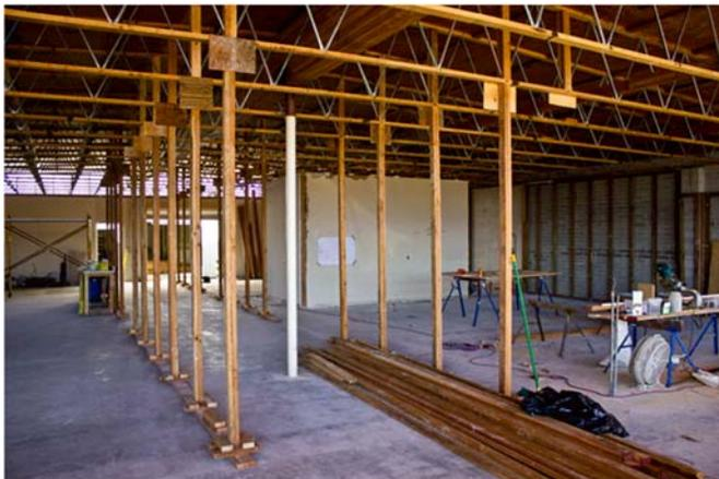
Richard & crew placed temporary supports through the center of the building before the roofing materials were delivered.
